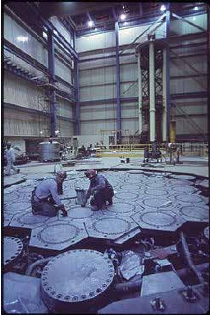
Fuel Loading Deck of the Fort. St. Vrain Core
