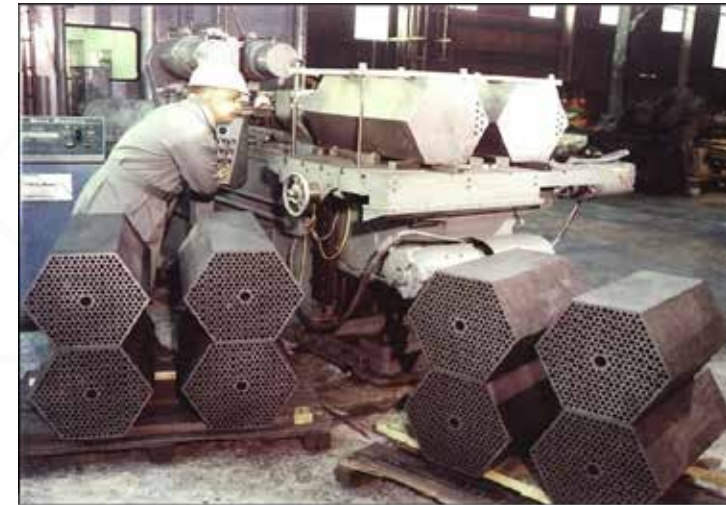
Gun drilling long holes in Ft. St. Vrain fuel elements Today - drilled with numerically controlled machines
